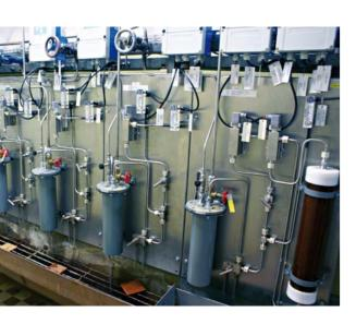
Panel for pressure and temperature adjustment of the samples in power engineering
