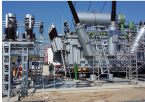
SS 400 kV Spišská Nová Ves power transformer 400/110 kV 250MVA
