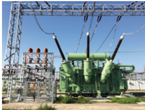
SS 400 kV Levice power transformer 400/110 kV 250MVA
