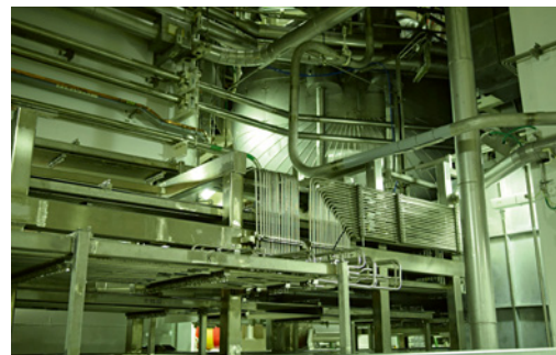
Steam generator and impulse tube lines of NPP Mochovce
