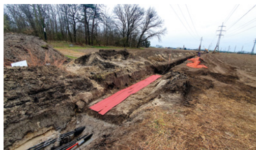
Excavation work and laying of HV cables – power station Stupava, power station Malacky
