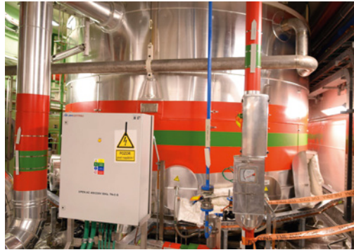
Tanks of emergency systems of NPP Mochovce
