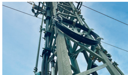
Transition of HV cable line to HV air line in the village of Lakšárska Nová Ves
