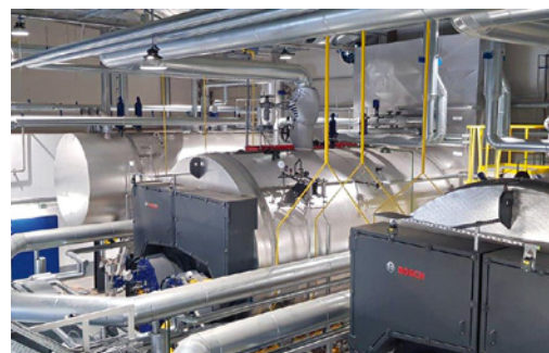
Steam boiler room in the heating plant of Slovenské cukrovary Sered'
