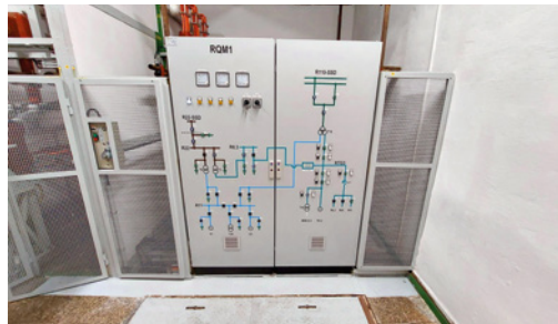
Control cabinet for generator outlet cell TG-3 Žilina
